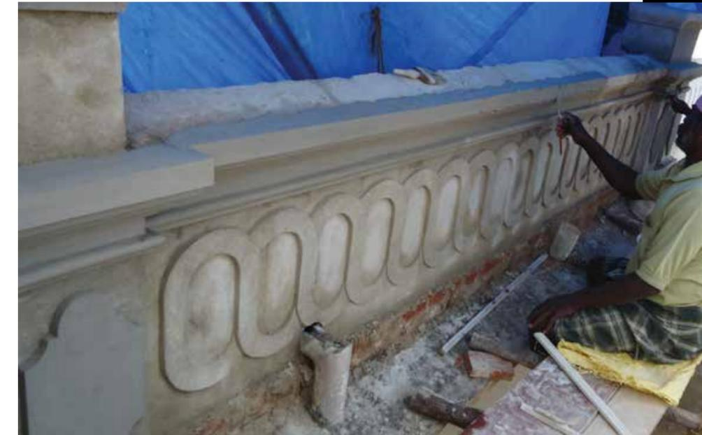
Ornamentation of parapet wall in lime mortar.
