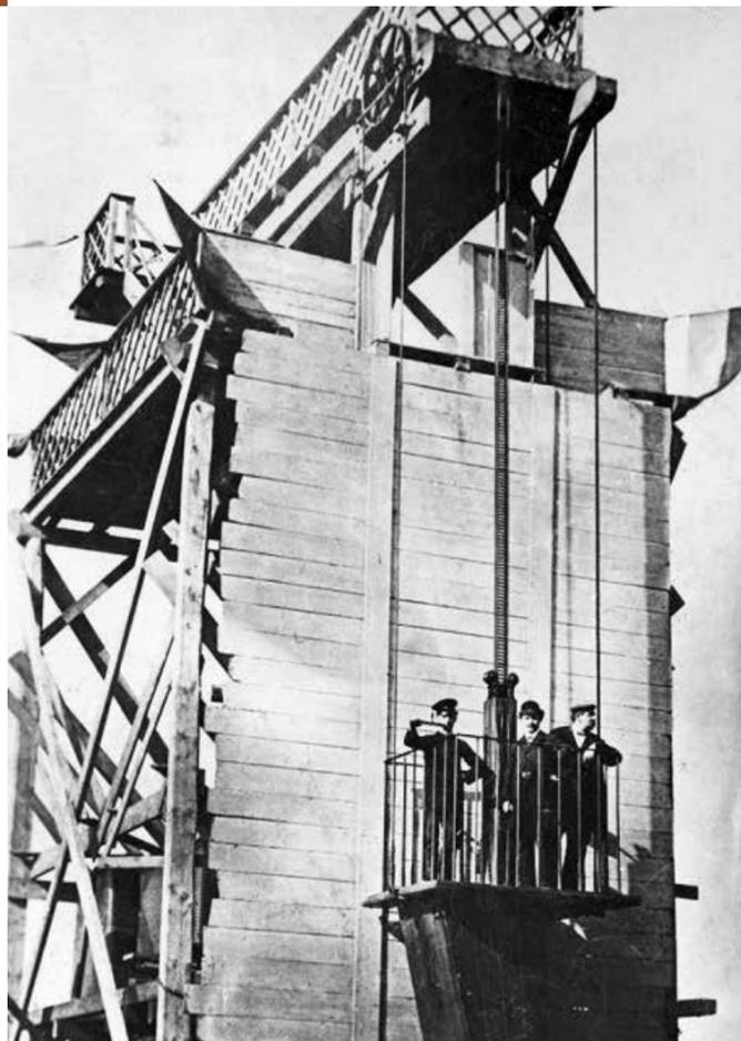
**Above:** Up 20 meters at 1.8 kilometers per hour – the first electric elevator at the Pfalzgau Exhibition in Mannheim, 1880. Developed by Werner von Siemens. Source: [new.siemens.com/](http://new.siemens.com/)
