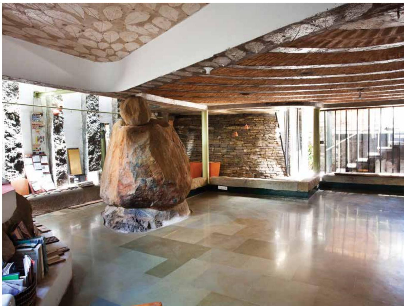
Brick ribbed slab ceiling and boulders found in the site incorporated into the basement.
