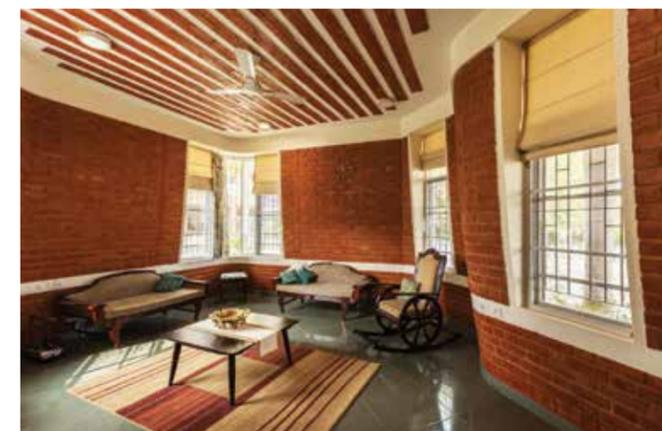
Brick filler slab ceiling complements the inwardly tapering brick walls.
