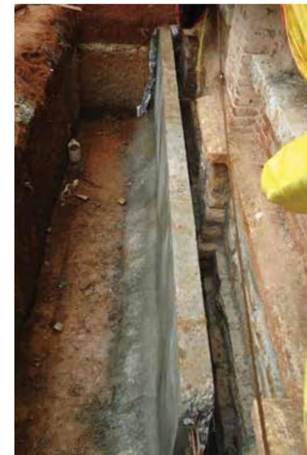
Diaphragm RCC to strengthen the foundation.
