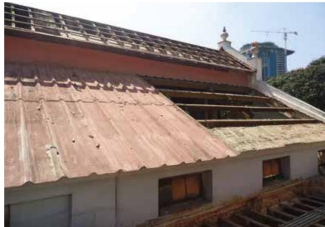
Existing Sloping Roof with asbestos sheets.
