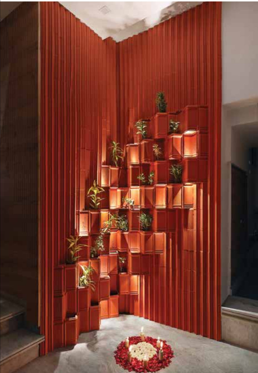
Clay roof tiles designed as planter boxes to create a mini vertical garden.
