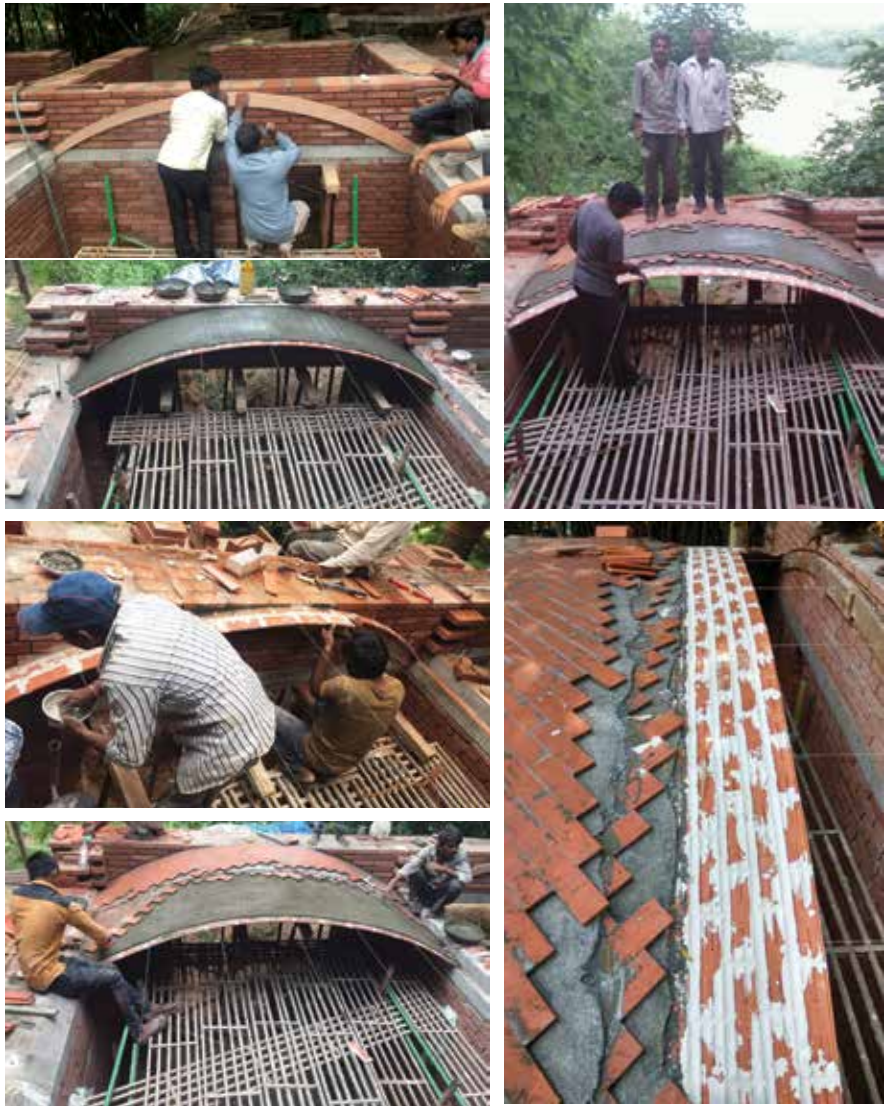
Timber vault construction in progress, Soach NGO, Ahmedabad.
