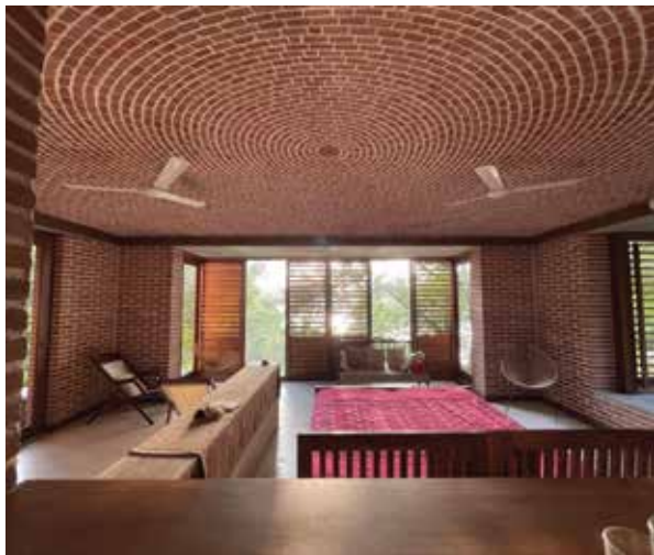
Rohtak dome and its construction process. Soach NGO, Ahmedabad..
