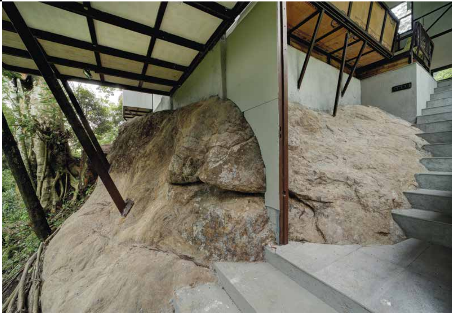
Steel directly bolted into the rock formation.
