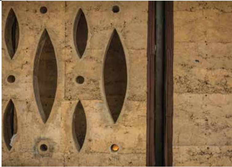
Walls constructed with debris, Bienalle Pavilion.
