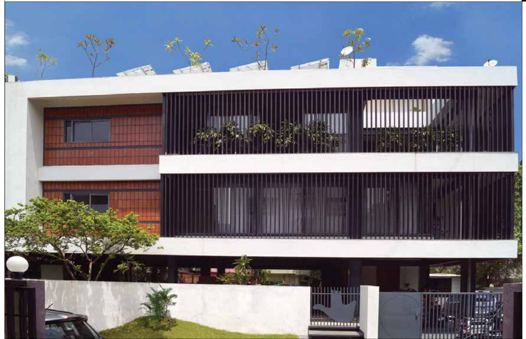
The facade displays an absence of lintels, overhangs, the walls built with clay blocks, the aluminium pivoted louvers bringing in dynamism – Heer Radha Residence.
