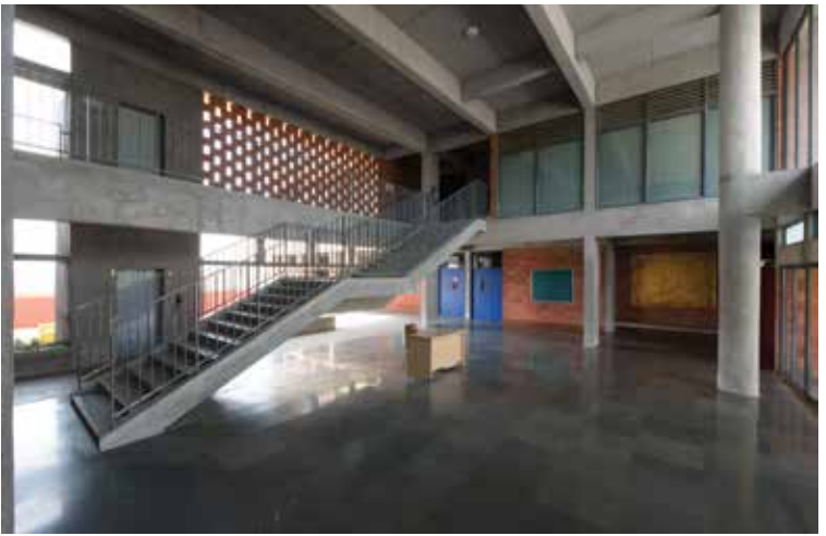
Exposed concrete, clay bricks, terracotta jaalis, rough Kota stone flooring articulate the building – Azim Premji Foundation, Yadgir.
