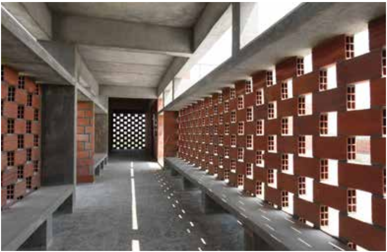
Hollow clay brick exterior walls cut the heat ingress – Azim Premji Foundation, Yadgir.
