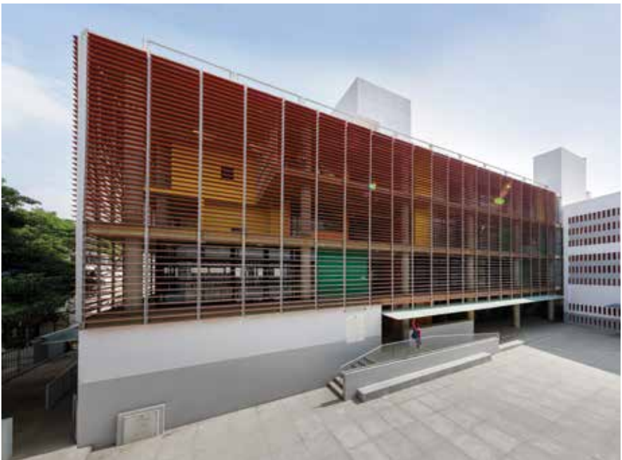
The double skin facade with the outer layer being bent steel louvers – Divya Shanthi Block.
