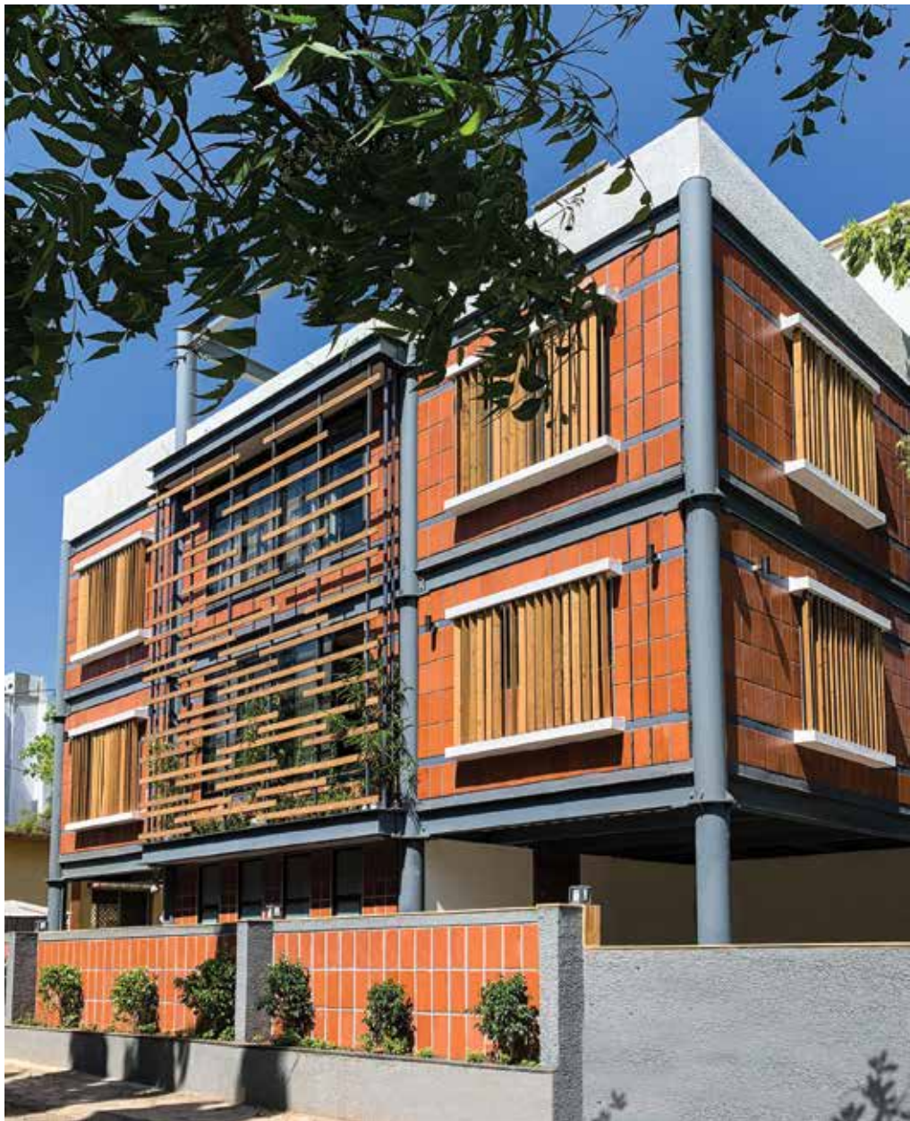
Circular steel columns, perforated clay blocks, vertical wooden louvered windows mark the elevation of the three level structure – Nuts and Bolts residence.
