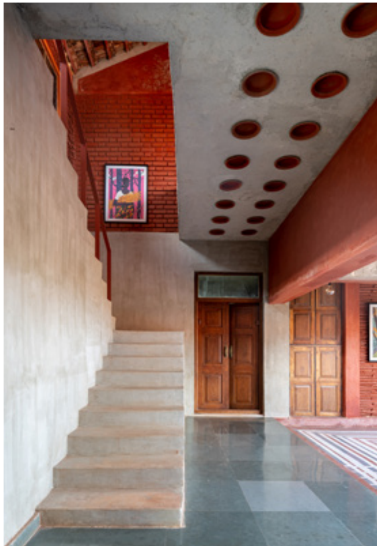
Green and grey Kota stone contrast the earthy hues of brick and terracotta filler slab roof
