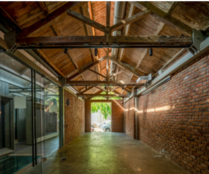
The thick plaster painstakingly scraped off to reveal the brickwork
