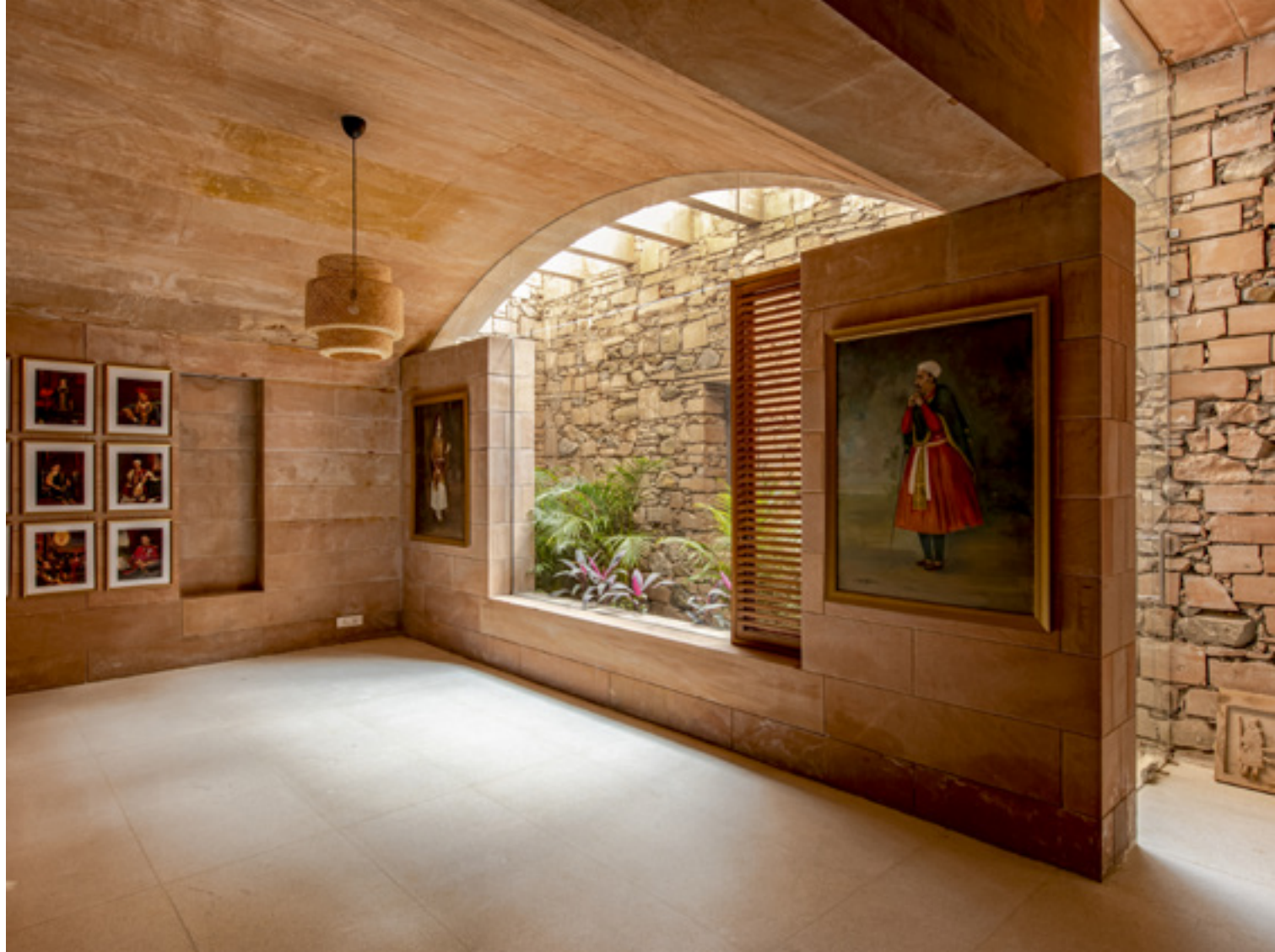
Courtyards, narrow slits, vaults, large single span stone pieces mark the structure
