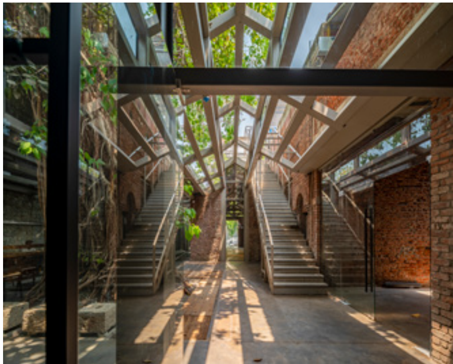
Glass ensconced openings created on the North light truss roof to let in ample natural light
