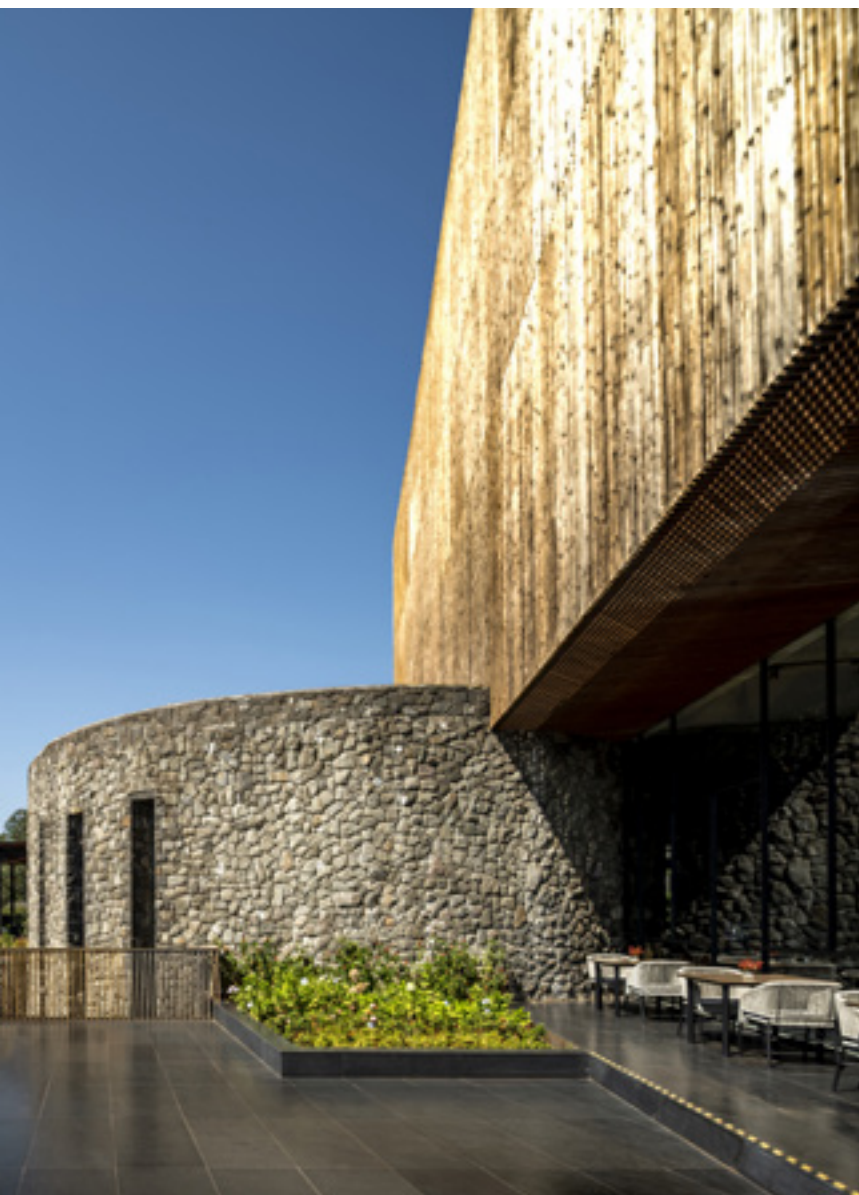
The load bearing stone masonry wall echoes the remains of an existing fort wall
