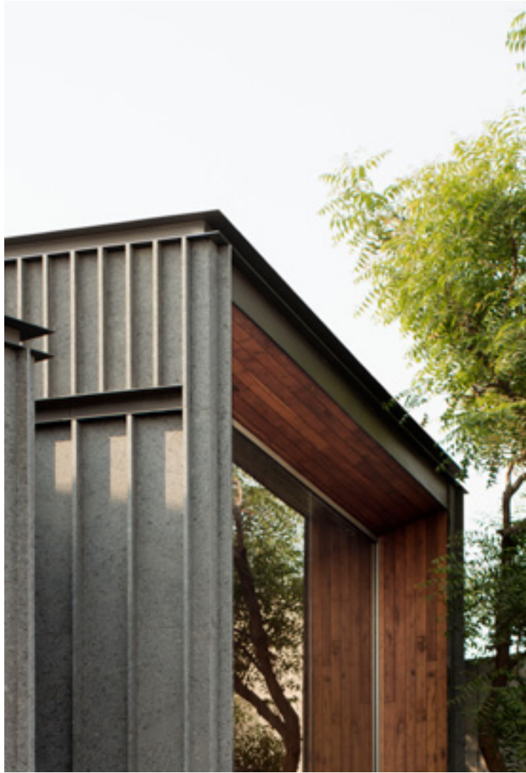
Light weight steel structure clad with thin ribs and slabs of local grey stone
