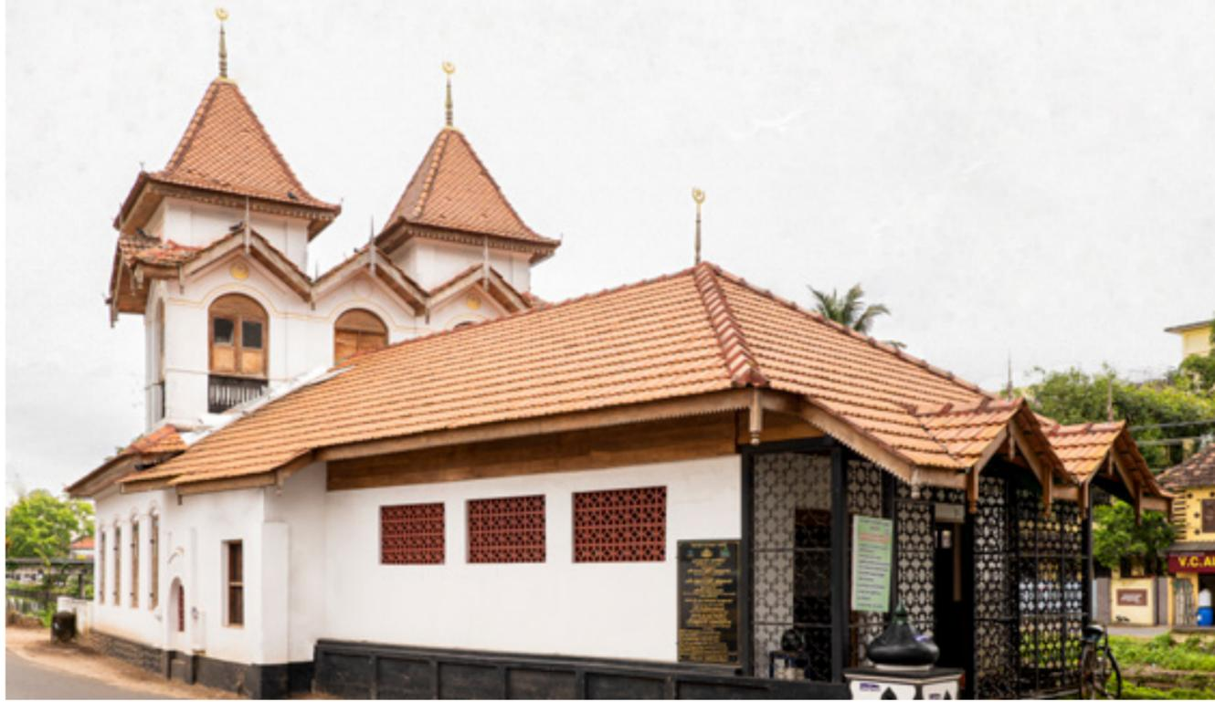
The asbestos roof added later in the Saukar Masjid was removed and replaced with the original form of clay tiles used in the core structure
