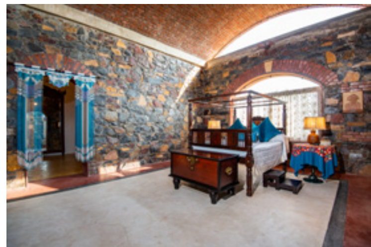
Jack arches, random rubble masonry lend the vernacular flavour in the bedroom
