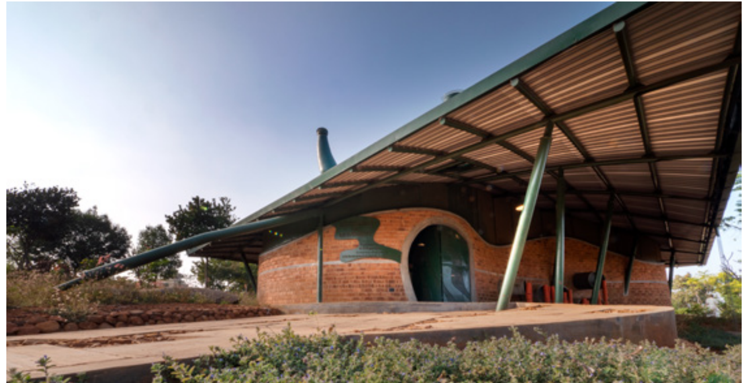
MS is bent three dimensionally to achieve the organic shape of the roof
