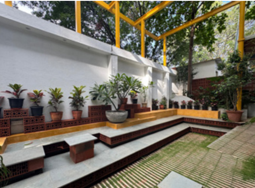
Informal gathering space defined with Kota stone seats over Porotherm blocks--Selco Foundation
