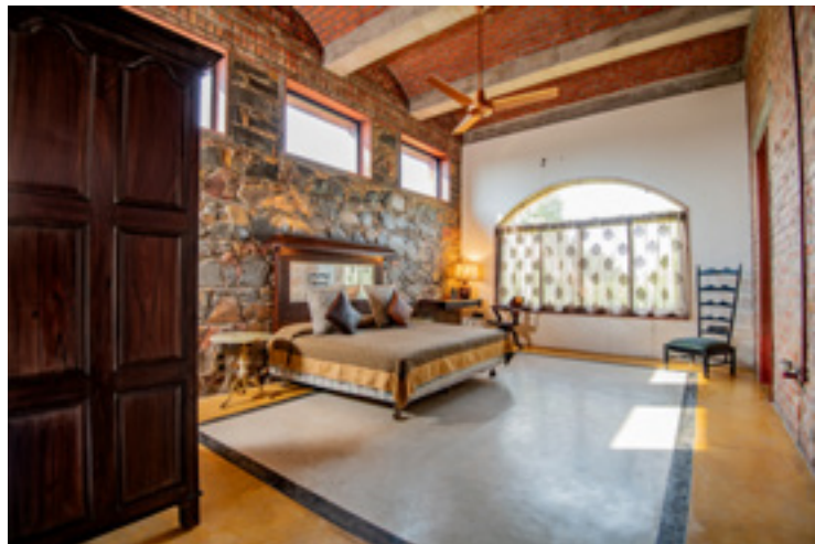
Random rubble masonry, brick vault, articulate the living area
