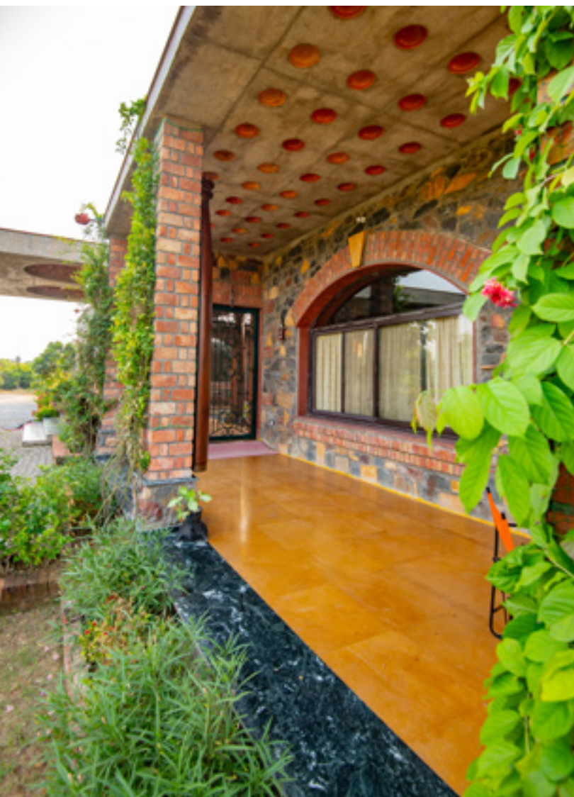
Large verandas, with filler slab roof, shade the interiors
