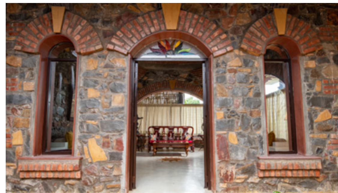
Entry is marked by brick arches and random rubble stone masonry
