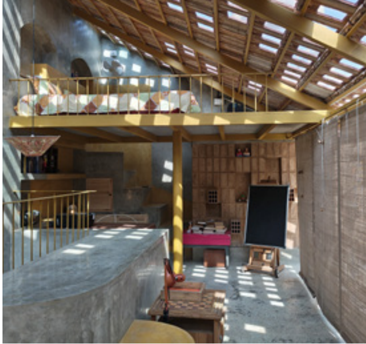
Tiled roof with light vents ushers in ample natural light--House of Thoughts
