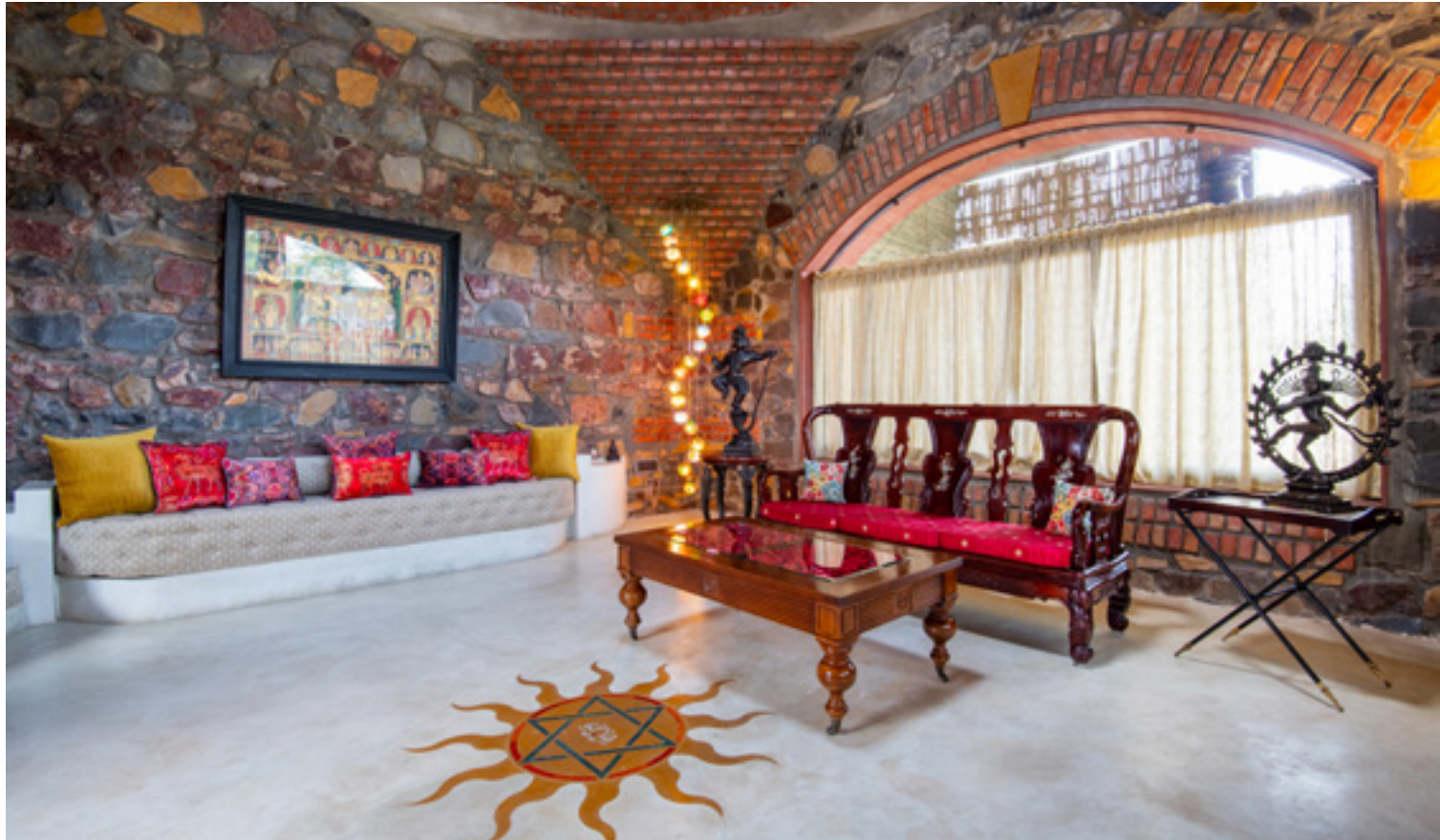
Random rubble masonry, brick vault, articulate the living area
