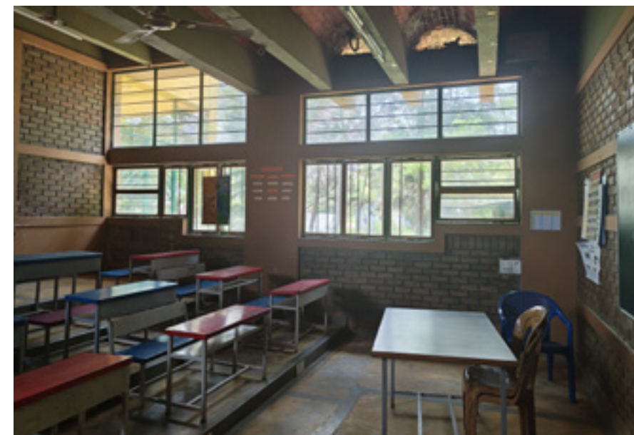
CSEB block structure with interlocking brick vaults and Jack arches--PSET School
