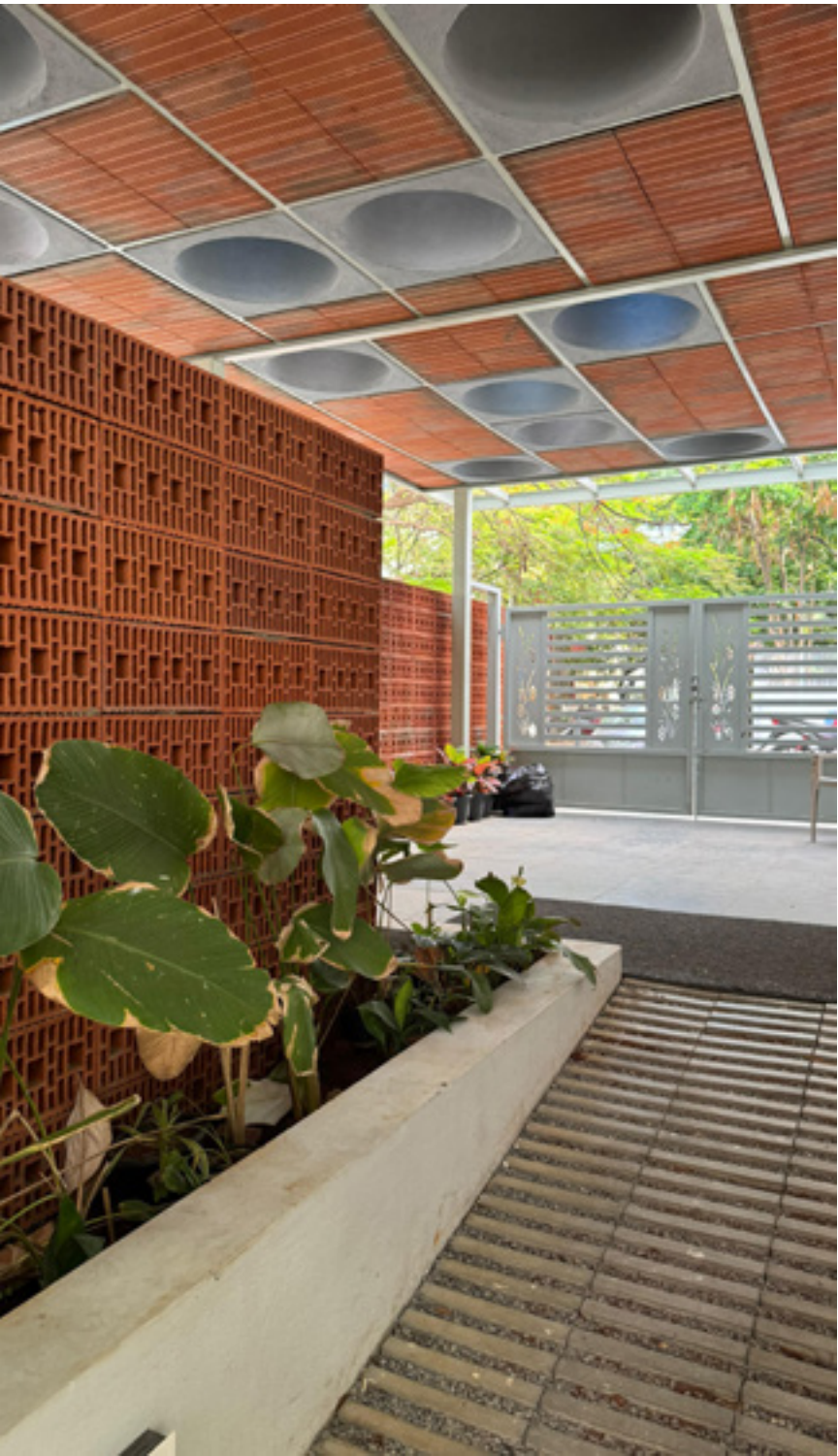
Roof over setback space with inverted terracotta pots--Selco Foundation
