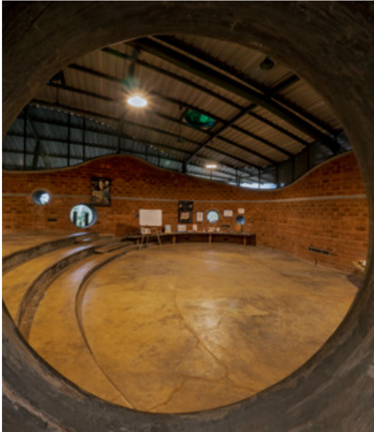
Apertures on the brick walls permit natural ventilation
