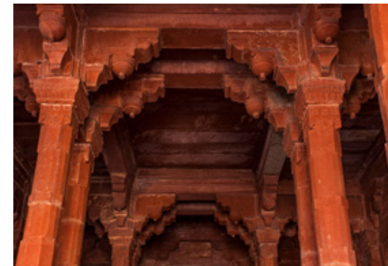
Example of trabeate and corbelled constructions in the mosque of Fatehpur Sikri IMAGE CREDIT : WIKI.
