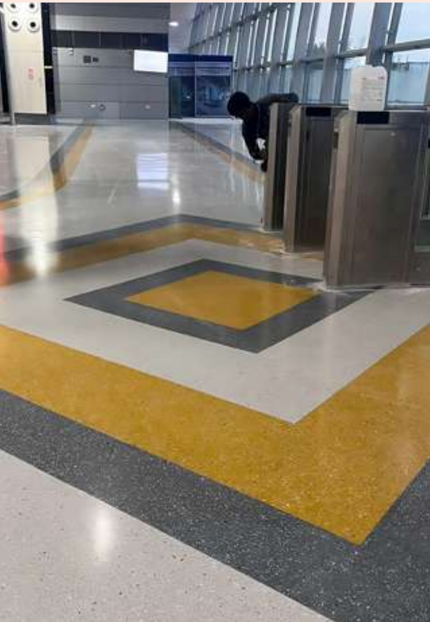
Terrazzo Flooring executed inside an airport
