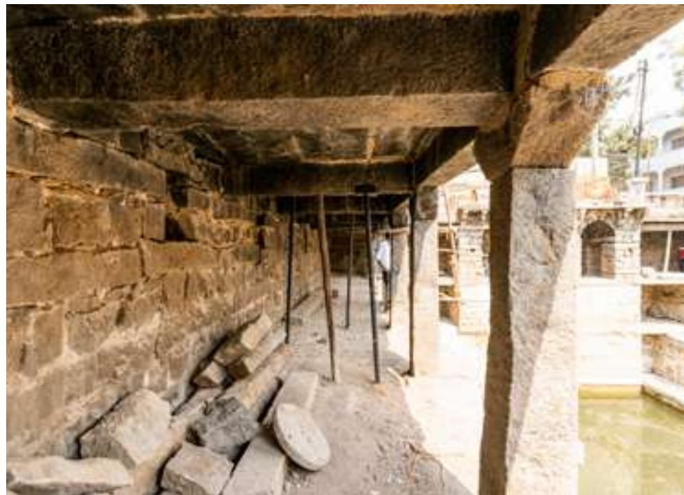
Rebuilding portions partly or fully damaged
