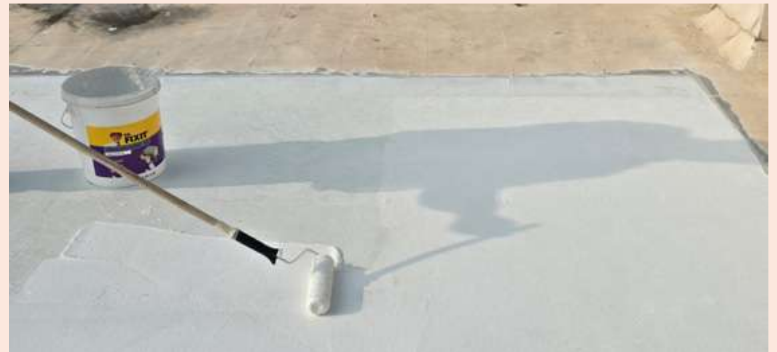
Wonderproof 100 application on exposed roof
