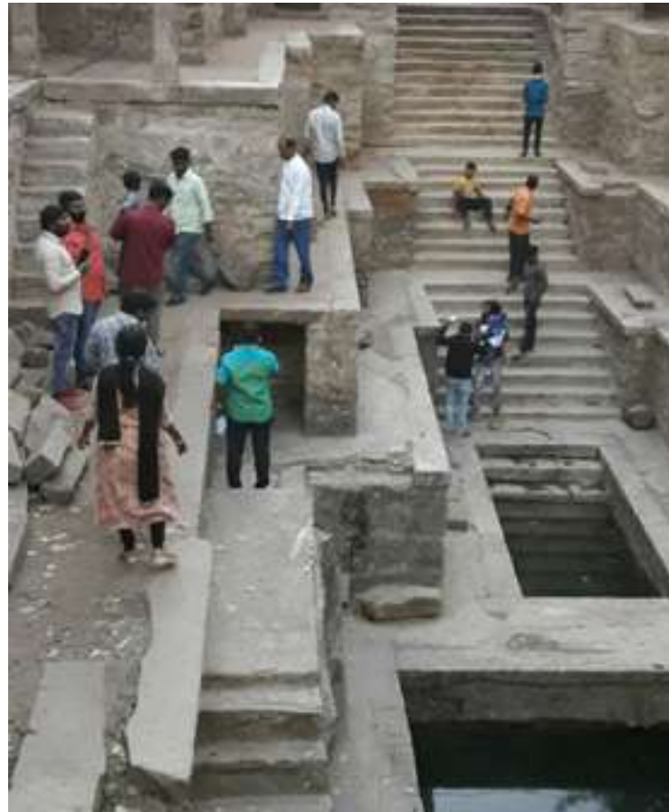
Work progress during restoration
