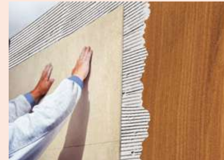
Application of Roff Masterfix
