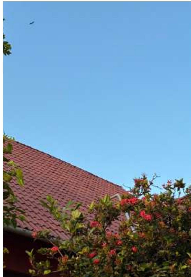
Polymer composite roof tiles manufactured using single use waste plastic
