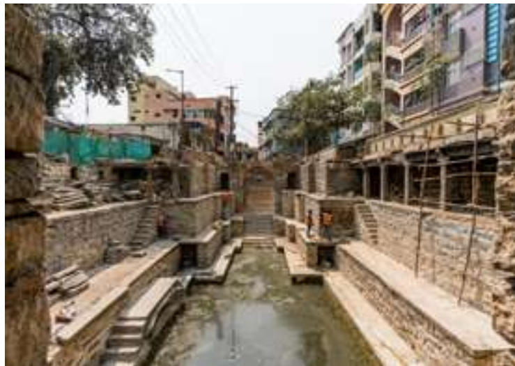
Strengthening, rebuilding the structural members
