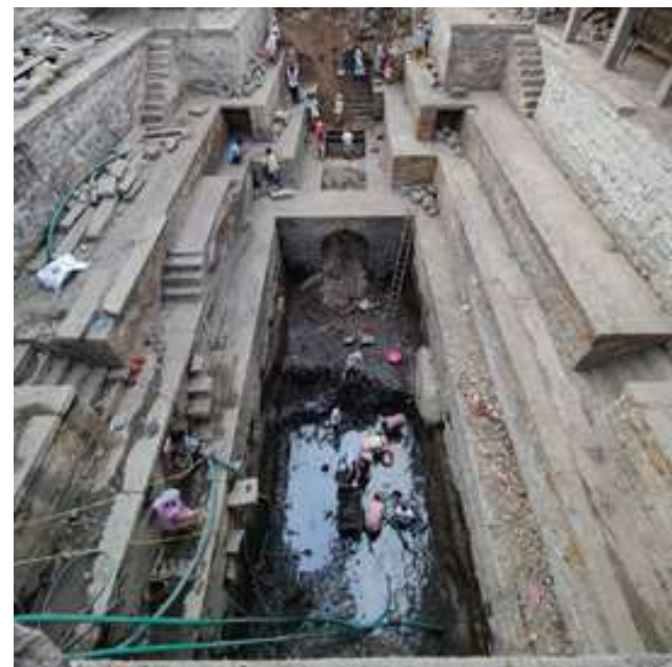
Capturing the ongoing restoration
