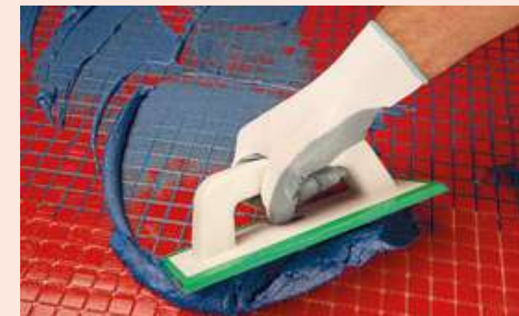
Roff Starlike used for tile grouting
