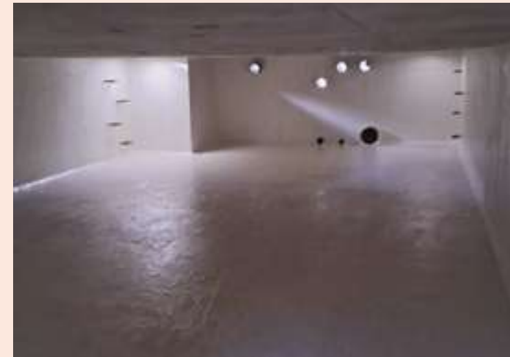
Dr Fixit Tank Pro application inside a tank
