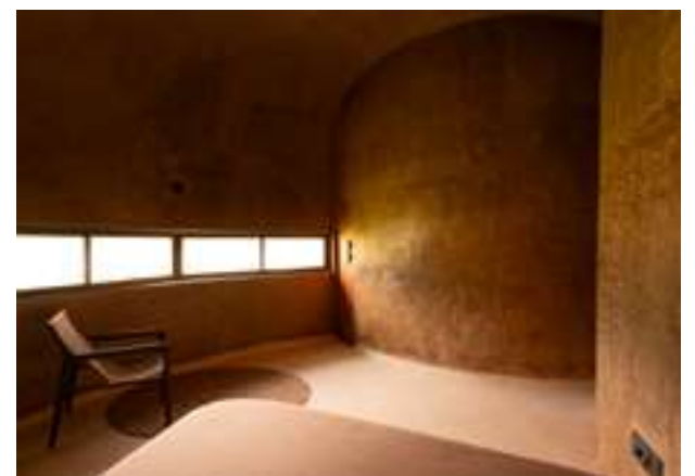
In-built furniture, structured in mud, mark the interiors
