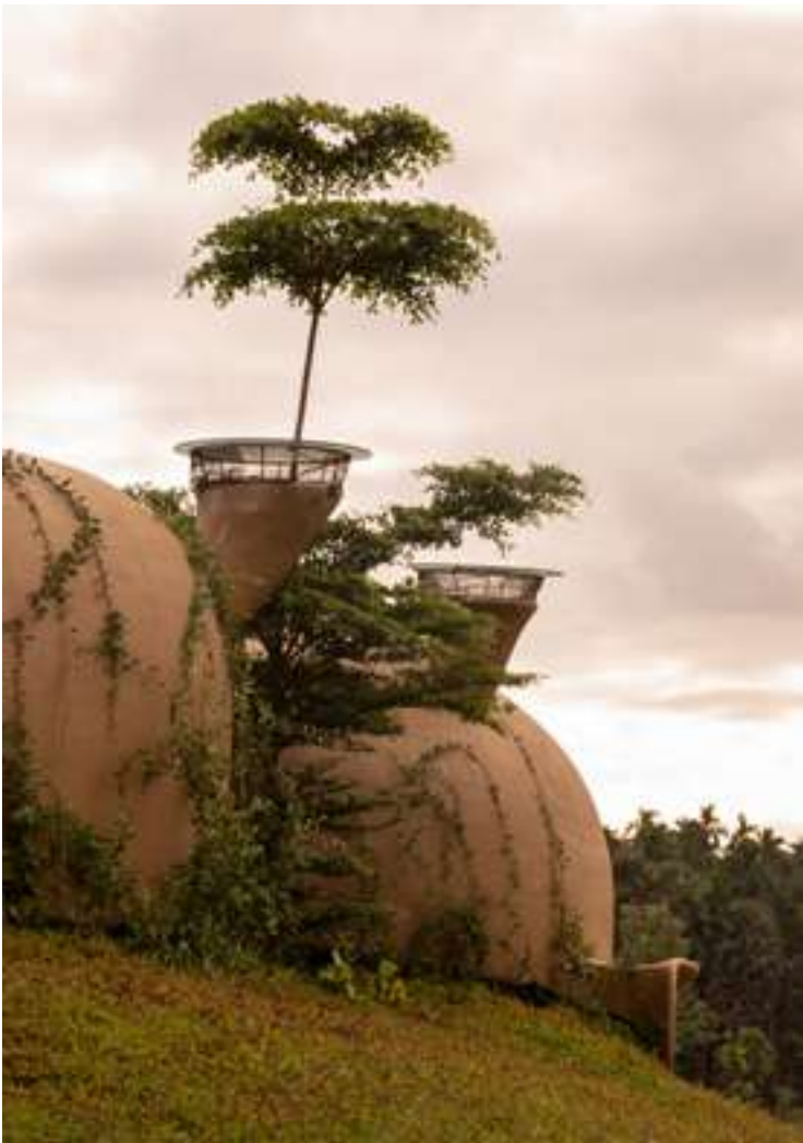
Funnel shaped hot air exit vents keep the interiors cool
