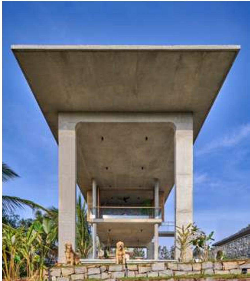
View of the cantilevered roof
